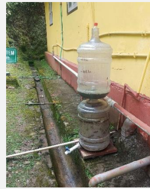
Karnataka model (effluent treatment) @ Damthang
